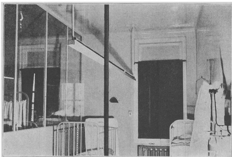
Fig. 5.—Room with ultraviolet irradiation of upper air.
